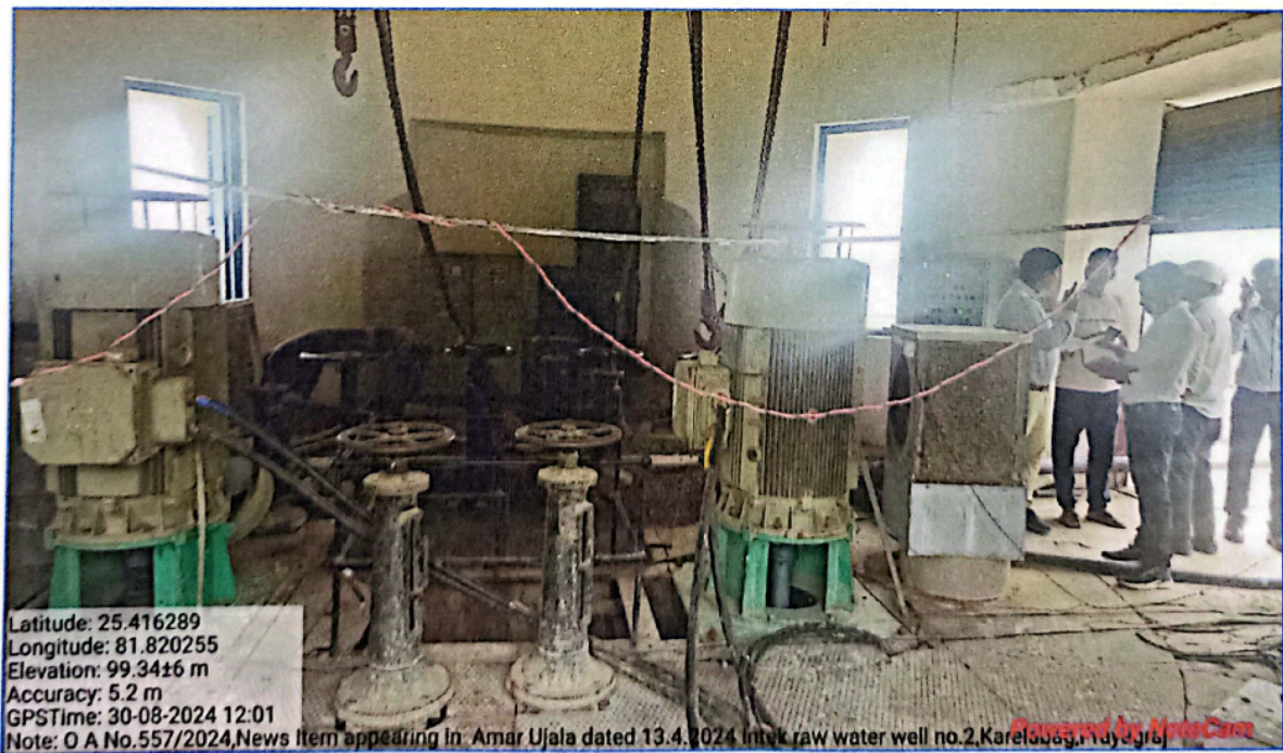
Photograph of Raw Water Intake Well No.2, Karelabagh Pumping Station, Prayagraj
